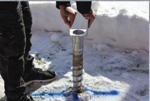
3. PLACE THE EARTH ANCHOR SCREW BY HAND THE FIRST STEP.
